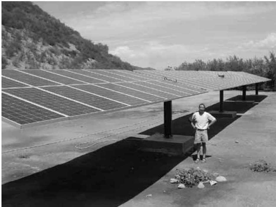
A 10kW single-axis tracking array, Jeff installed at Glen Ivy Community in Corona, California.
