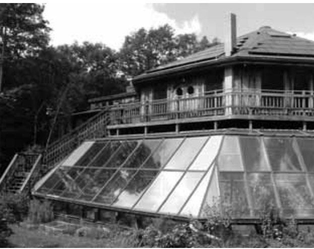
The Common House at Sirius Community in Shutesbury, Massachusetts, USA employs a passive solar greenhouse, solar hot water, as well as triangular solar electric modules on the octagon roof.
