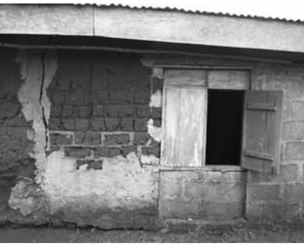
Close-up of sequence above. (As repairs became necessary, the latest materials and techniques were used).
