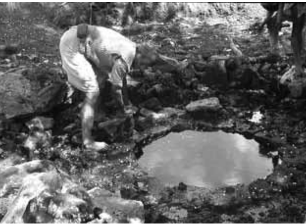
Non-cement water tank filled with water, which will now be covered with a wooden trap door.
